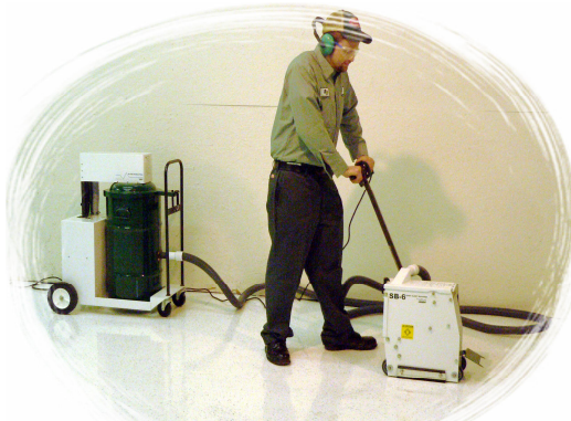
Attached to the SB-6 Shotblaster with 1.5+Hose
